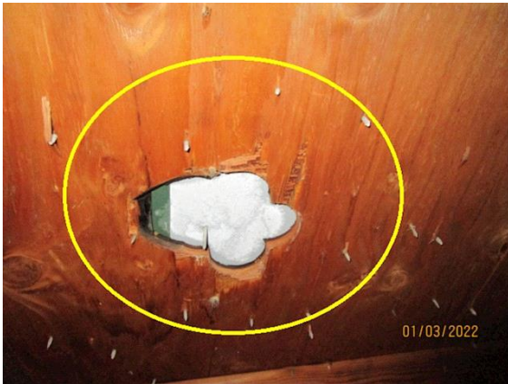
Attic / Roof Framing and Sheathing:
