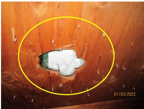
ATTIC / ROOF FRAMING AND SHEATHING:
