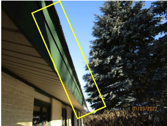
ROOF DRAINAGE SYSTEM:
