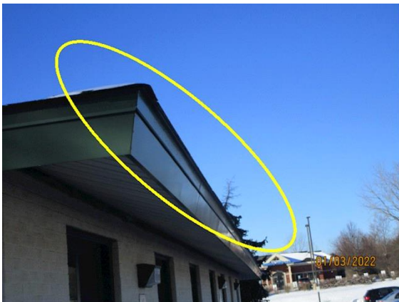
Roof Drainage System:
