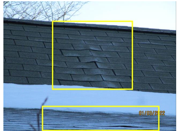
Roofing: Uneven
