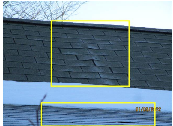
ROOFING: Uneven
