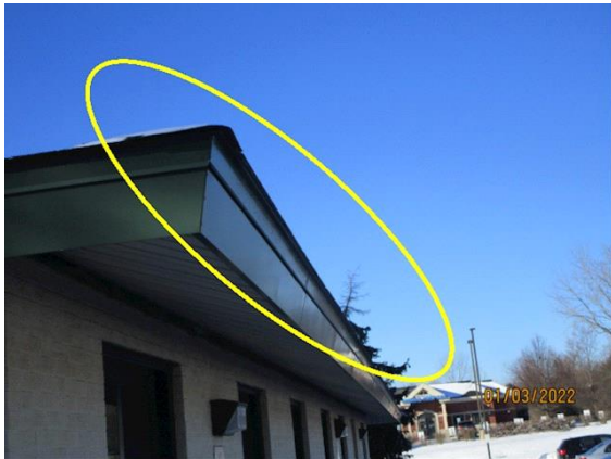
ROOF DRAINAGE SYSTEM:
