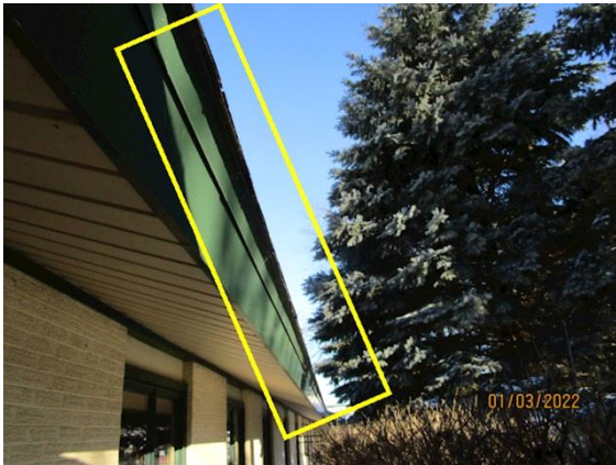
Roof Drainage System:
