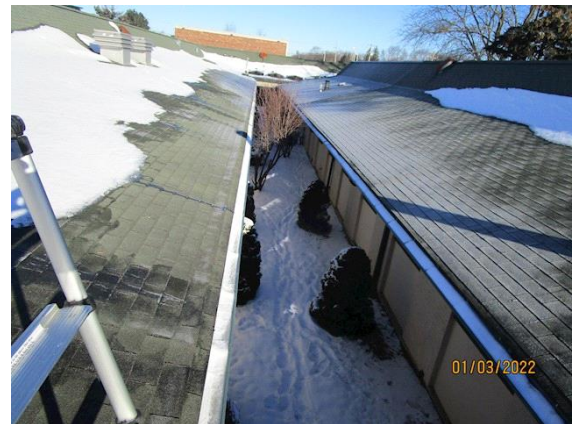
Roof Drainage System:
