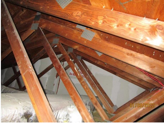
Attic / Roof Framing and Sheathing:
