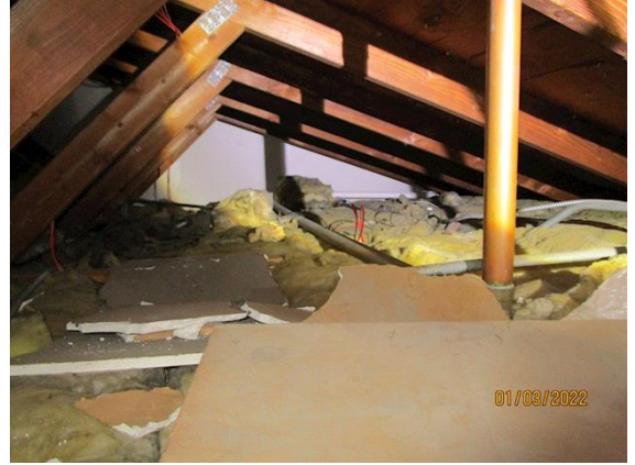
Attic / Roof Framing and Sheathing:
