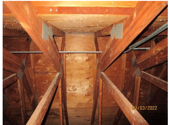
Attic / Roof Framing and Sheathing:
